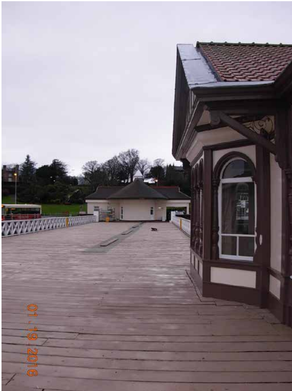
Southern Arm of Pier – January 2016. Note the gaps between the decking boards have been closed up, joints between boards have been staggered, surface is now more level, antislip treatment has been applied across the full width of the deck and handrails have been refurbished.
