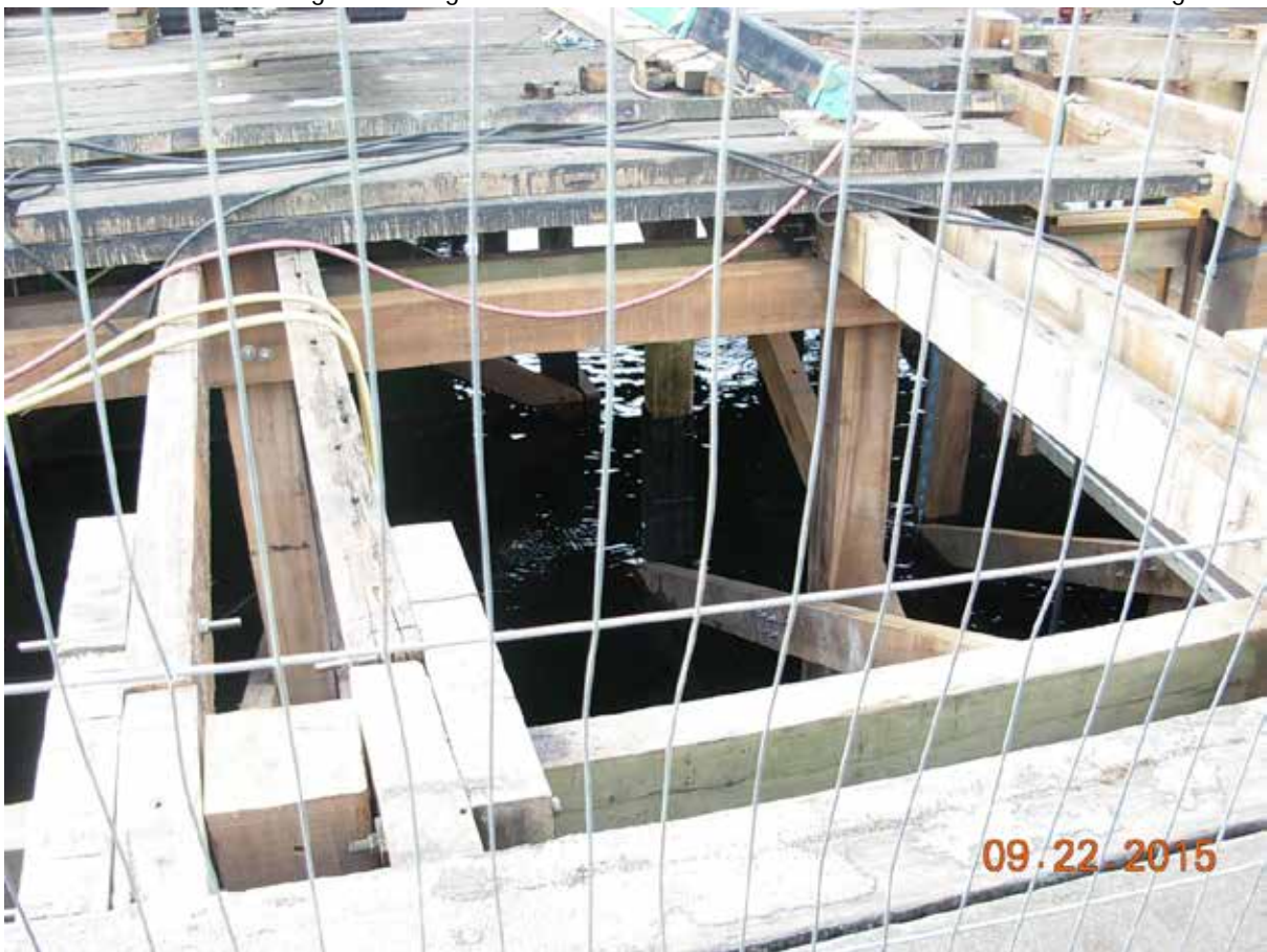
Structure of Pier – note replacement timber columns, ties and braces
