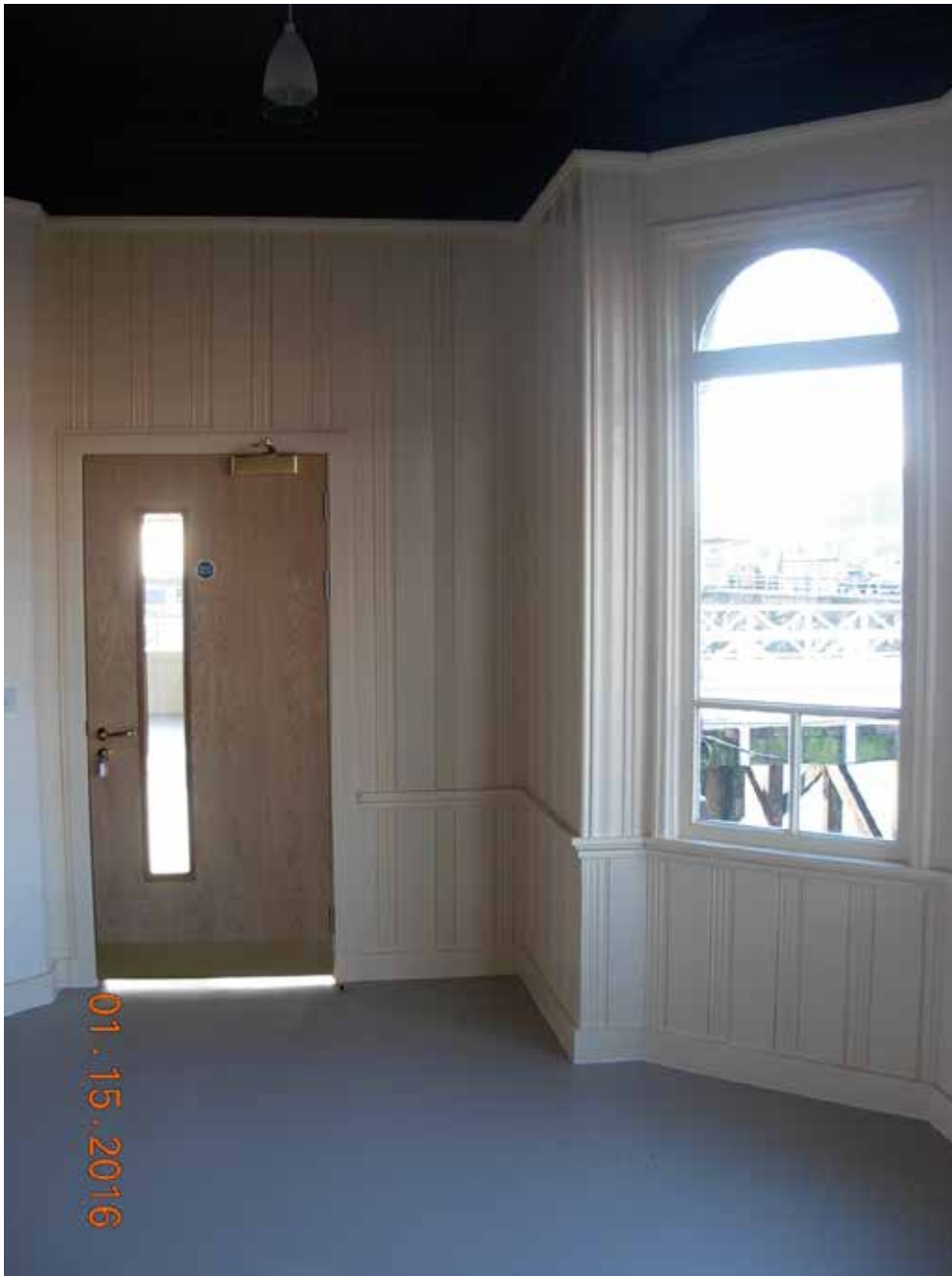
Ground Floor Entrance Lobby: tea-prep facility on the right hand side and new access into the First Class Waiting Room
