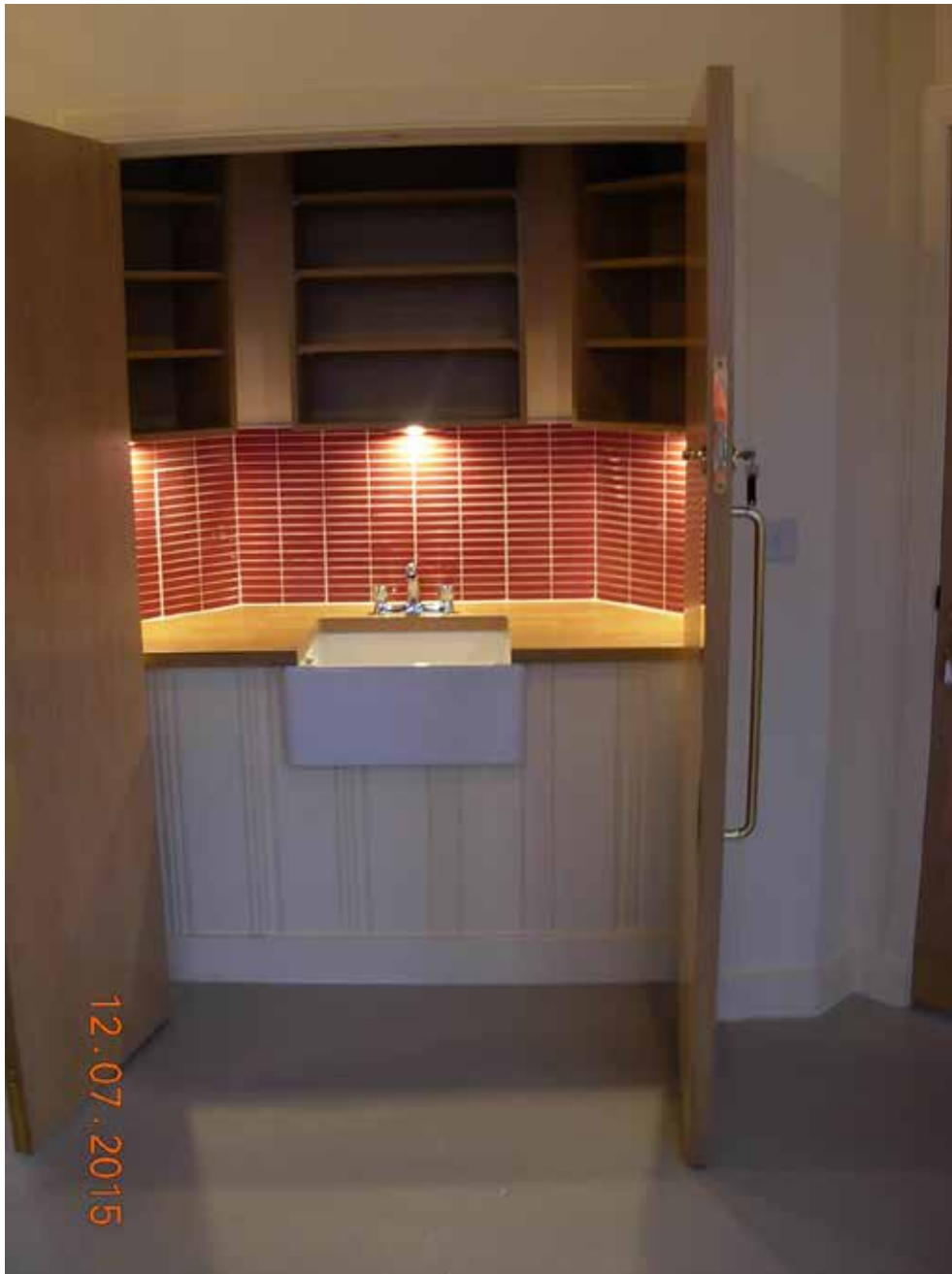
Ground Floor Entrance Lobby – creation of tea-prep facility to service the multi function rooms on the ground floor
